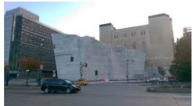
Award winning Salt Storage Building NY
