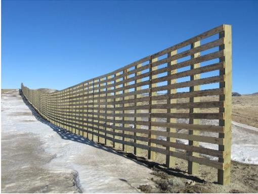
Although not the earliest use of vertical fence in the state, starting in 2008, the Wyoming Department of Transportation started building vertical fences. WYDOT has built three types of vertical fence: wood face boards on wood posts, polymer strap on steel I-beam, and polymer strap on 12" round posts. These fences are 6 to 12 feet tall depending on placement. While they can be expensive to build, maintenance is reduced due to the lack of anchor failures.
